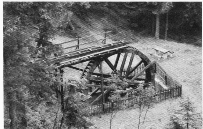
Waterwheel driving Fahrkunst (man-engine)
